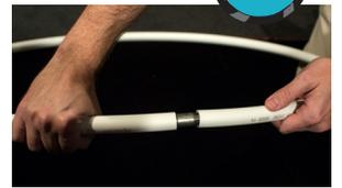
Slide on the other end of the tube until both ends meet.
